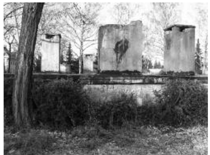
Bunker Bundesring Nord
